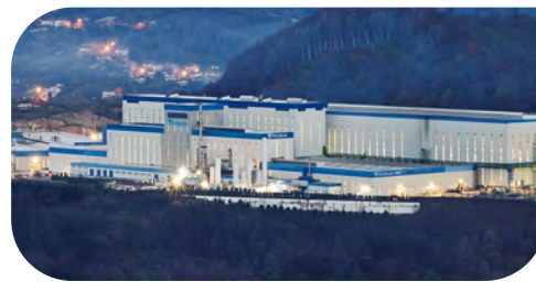
Establishment of the TATMETAL Facility
