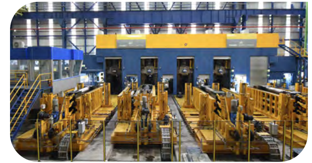
PLTCM Phase 2 - Continuous Pickling Tandem Line
